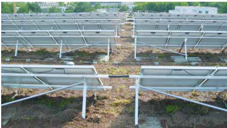
Tittmann Solar | State Theatre Stuttgart - Germany System: 112 kW | Triangle System
